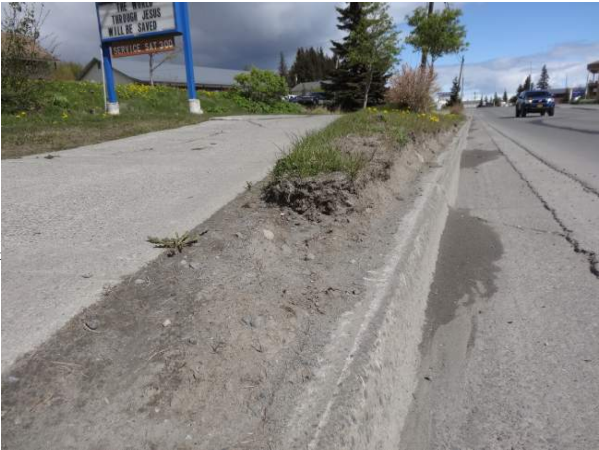
Pics of raised sod between Curb and sidewalk in front of 7th Day Adventist Church at 210 E. Pioneer
