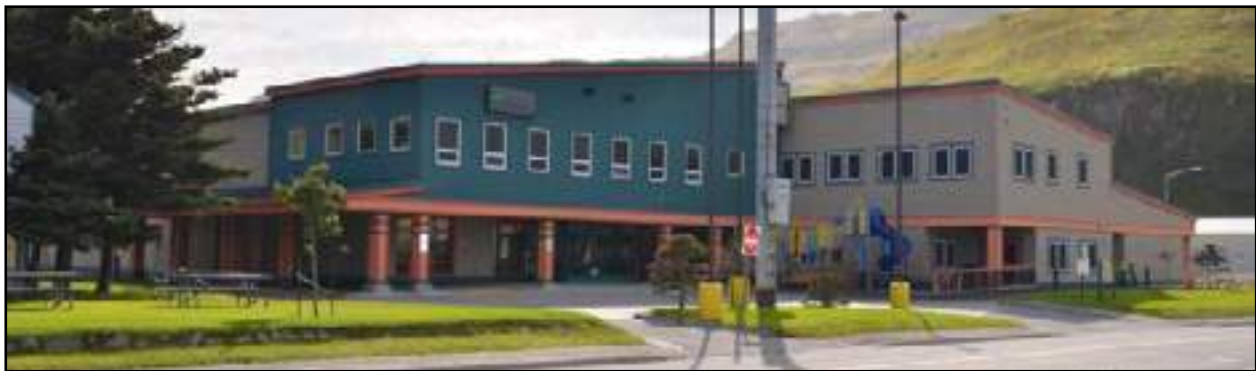
The City of Unalaska’s Community Center is the hub of community activities. Centrally located, the Community Center is widely used by both residents and visitors. It has everything from a cardio and weight room to music and art areas.
