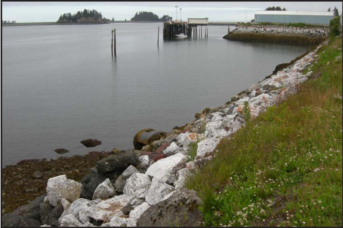
Figure 2. Most of Main Street and the Seldovia shoreline was extensively filled and rip-rapped by the U.S. Army Corps of Engineers after the 1964 earthquake. Note depth of fill and old cannery boiler.
