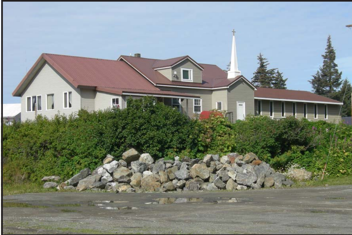
SEL-331 (Springer's #1). The narrow central block of the Seldovia Bible Chapel "was built in 1944 by Rev. George Tobleman and reputed to have the strongest concrete in town." The north (right) wing was built in the 1970s, the south (left wing) was added later.
