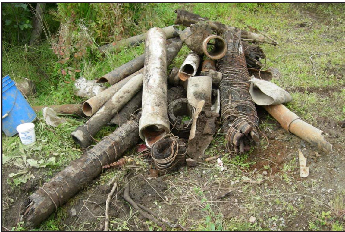
Figure 30. Wood-stave and metal pipe of various diameters was removed from beneath English Road.
