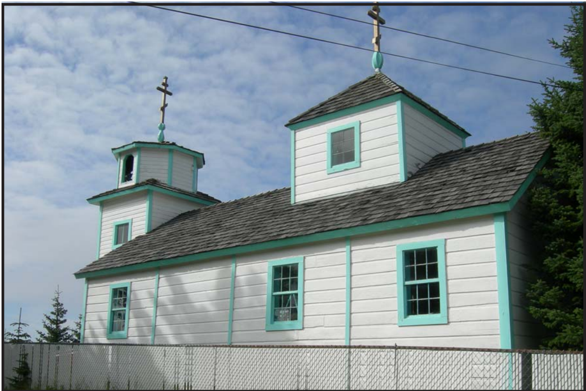
SEL-023. Most of the Russian Orthodox church was built by 1891; the front tower was added by 1906.
