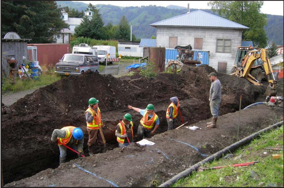
Figure 20. When an 18"-thick historic midden was found beneath English Road, construction crew members helped recover artifacts using hand tools. The old hospital (SEL-335) is at upper right.
