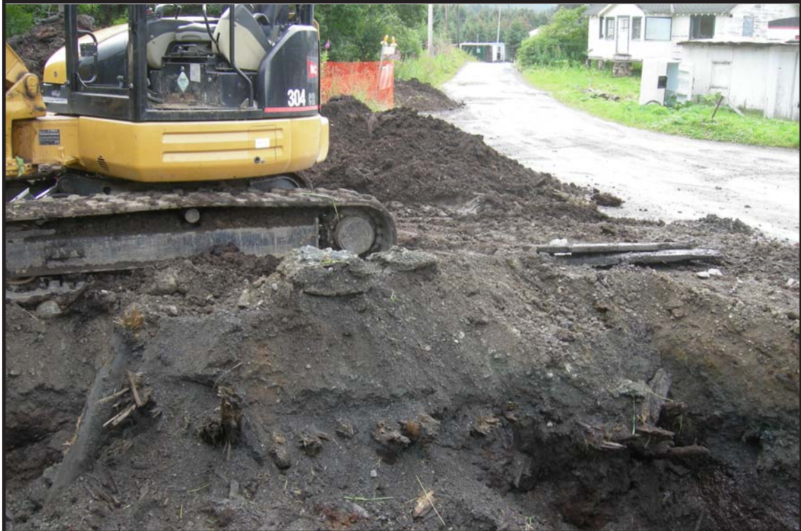
Figure 21. Excavations at the intersection of English Road and Alder Street (here looking southeast down Alder Street) revealed a pavement of parallel logs -- the remains of a corduroy road built to support vehicles traveling over the soft muskeg. The white house at far upper right is SEL-344.
