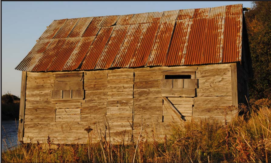
KEN-561 -- A log cabin on pilings by the river at the north corner of the village, composed of many short hewn logs butted end-to-end, is called the Creole Cabin and was built by John Astergin in about 1903 according to the AHRs form for KEN-060 (the building was inadvertently assigned a second number).
