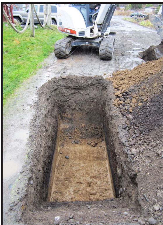
Figure 135. Trench 29, here looking southeast, was located near the intersection of Mission Avenue and Hillcrest Avenue.
