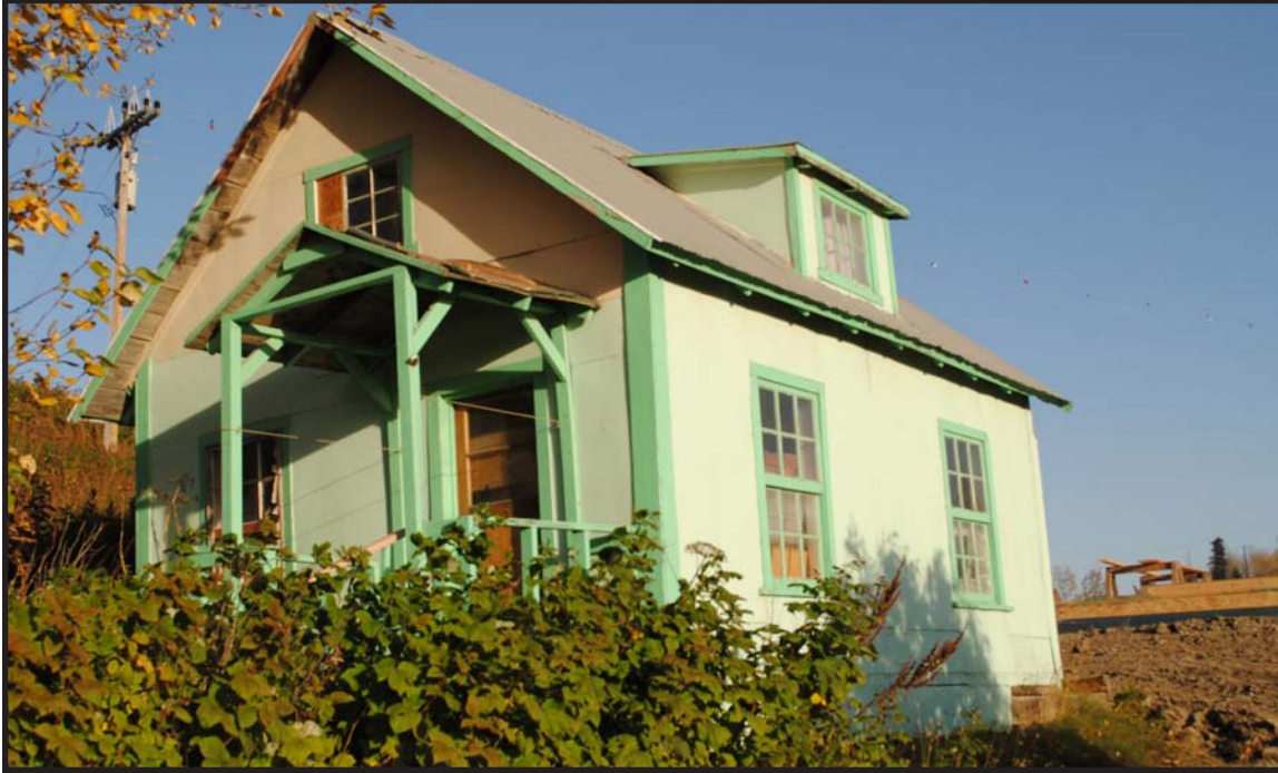
KEN-556 -- This green house with 6/6 double-sash windows is remembered as Nadia Oskolkoff's house, and is said to be a log building beneath the milled siding. Lascy (1904) plotted the building on USS 367. Here viewed east, in 2010, the building partly hides the pad for the new Russian Orthodox church rectory at right.
