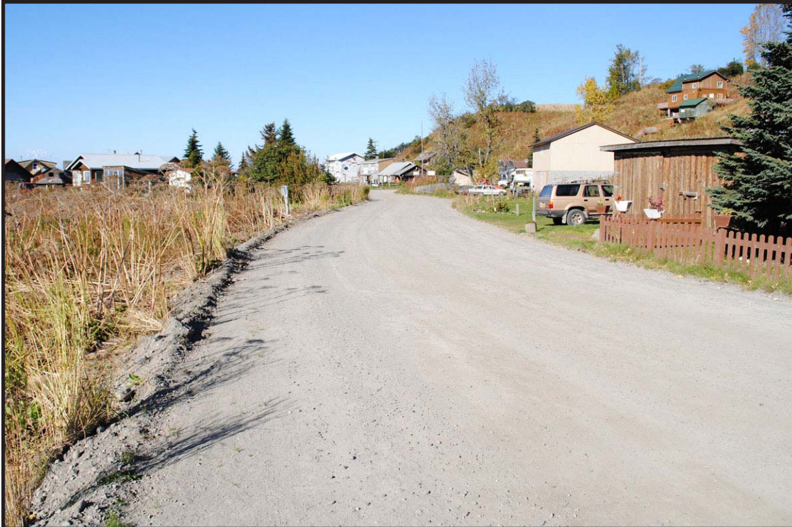
Figure 34. Mission Avenue, here looking northwest, appears to be mostly gravel fill over what was thought to be possibly a former land surface.
