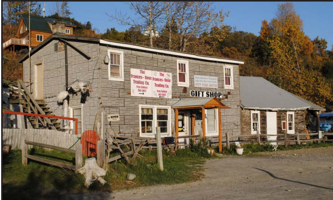
KEN-218 -- the Frances-Rose store, looking east. According to the AHRS form, the composite building first consisted of a one-story log cabin built by John Astergin in the 1880s, and is also known as the Astergin-Cooper-Churkin-Kraskoff house. Later another one-story log addition with dovetailed joints was built on the east, and then three frame additions -- two two-story -- were built on the west and north. The building is currently home to Laura Trunnell.
