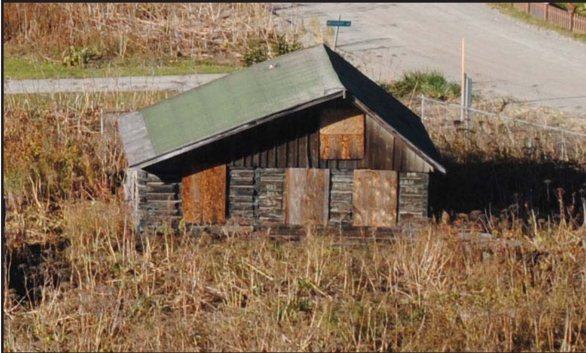
KEN-557 -- Here viewed northwest in 2010, the Jackinsky cabin still displayed numbered logs showing how the building components were numbered, disassembled, and reassembled closer to Mission Avenue with the axis shifted 180 degrees. A 1952 photograph shows the building with the shorter roof facing left, towards the southwest.
