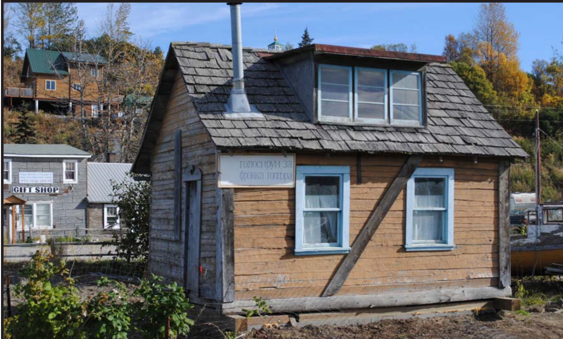
KEN-553 -- This log cabin (here looking northeast) was reportedly moved to Ninilchik from somewhere else and placed on a newly graded site in about 2009-2010. Some residents call it "Chaika's Roost." The sign on the building reportedly says "Vote for Frank Tupper" in Cyrillic.
