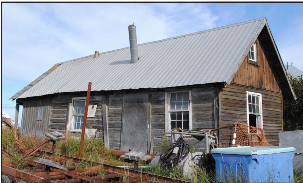
KEN-551 -- A cabin with logs hewn square, here looking north-northeast in 2010, shows in the same location in two of Alyce Anderson's 1911-1918 photographs. By 2012 the building had been removed and relocated out of the old village.
