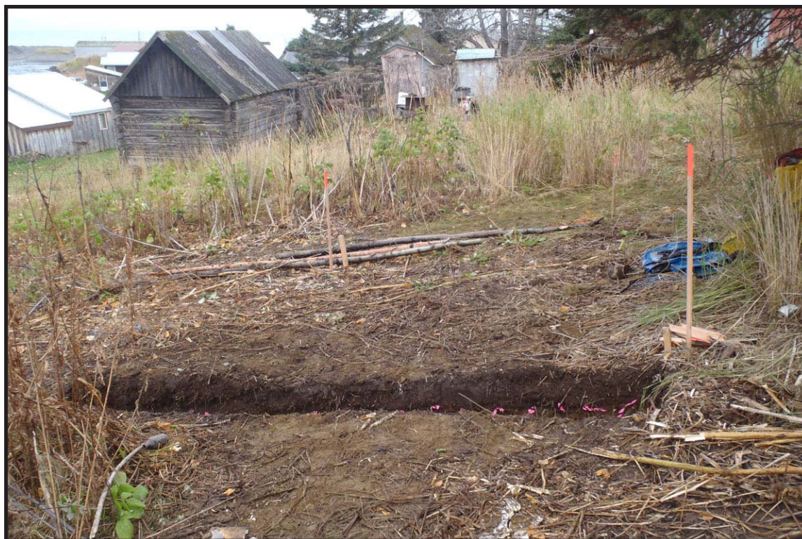
Figure 152. Trench 48 (here looking west) was dug with hand tools up Missionary Way NE. The old Russian Orthodox church school (KEN-031) is at upper left.
