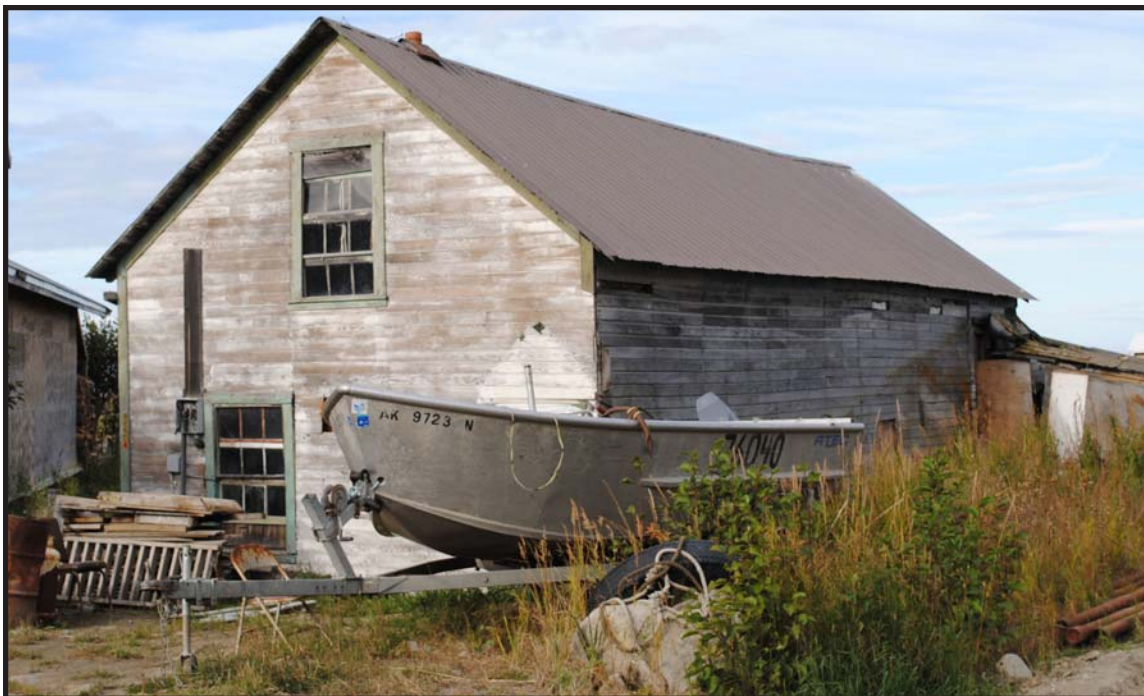
KEN-550 -- A large 1.5-story frame building located at the end of Mission Avenue, where the bridge used to go across the creek, shows in a 1911-1918 photograph. At that time a shed-roofed block extended across the entire north wall; a remnant of it remains at far right. At various times the building served as a dance hall, pool hall, and post office. Windows are 6/6 double-sashed wood examples.
