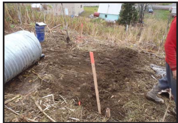
Figure 159. Trench 53 (backfilled, right of center, looking south) was dug using hand tools at the top of Missionary Way NE. Hillcrest Avenue is at the back of the photographer; log cabin KEN-560 is immediately to the right, out of the image.
