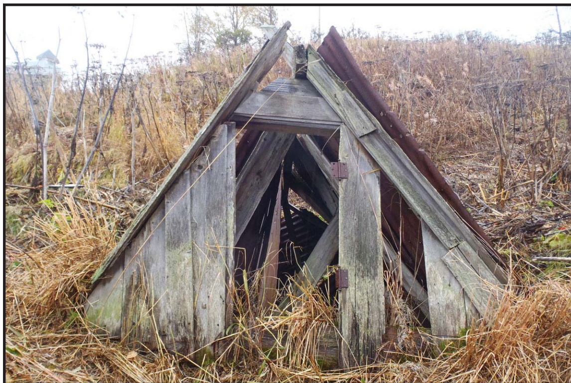
Figure 99. One of the two root cellars comprising KEN-555 still has a gabled portion showing, over the dug-out portion beneath.
