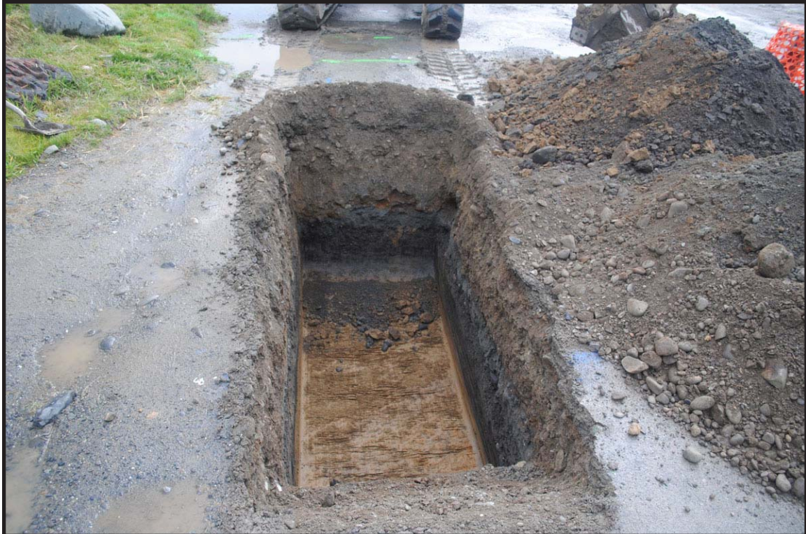
Figure 137. Trench 30 (here looking southeast) was dug with the machine at the northwest end of Mission Avenue
