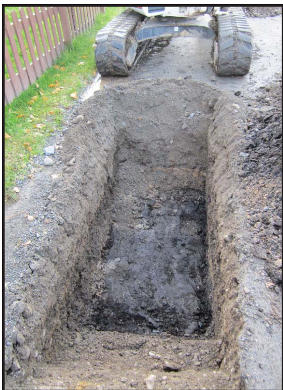
Figure 125. Trench 15 was dug in the roadway of Mission Avenue, in front of Deanna Smith's picket fence. View is southwest.
