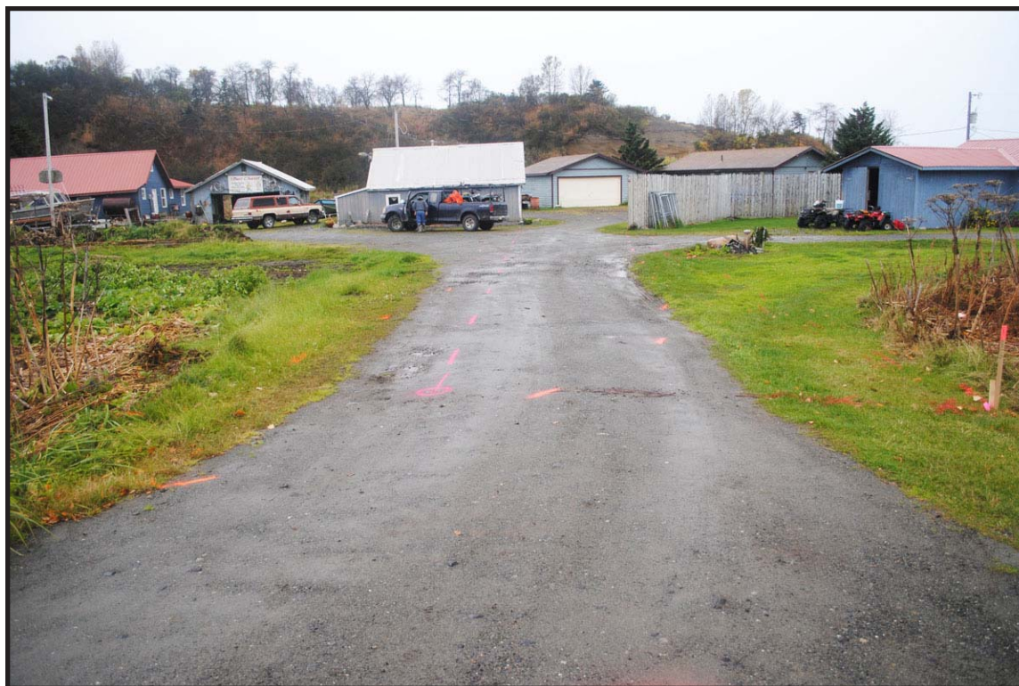
Figure 116. Four trenches (11 through 14) were excavated by machine among the buried utilities and property lines shown here painted on the ground in this view southwest down Missionary Way SW. Trench 11 was dug at extreme lower right.
