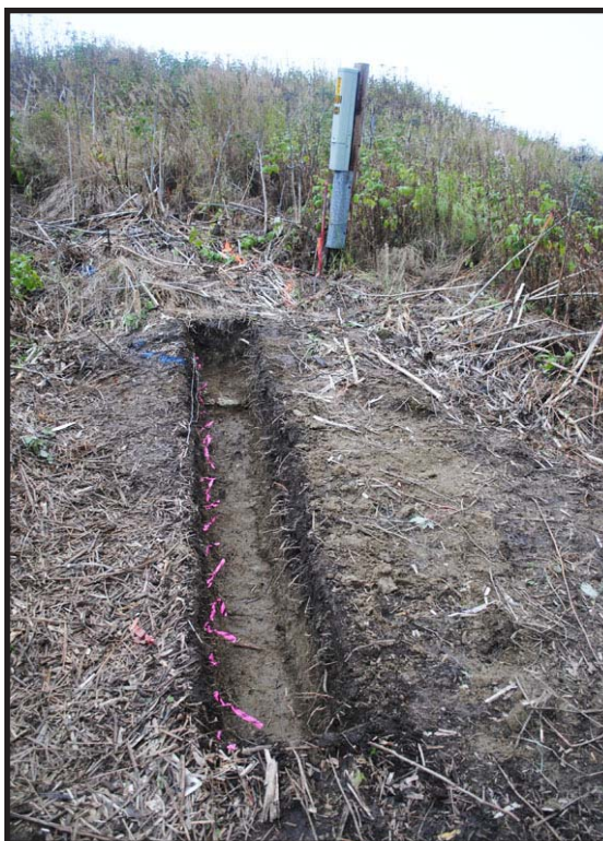
Figure 61. Upslope from Trench 50 (foreground, looking northeast) the grade steepened, and consequently Trenches 51-52 were not dug.
