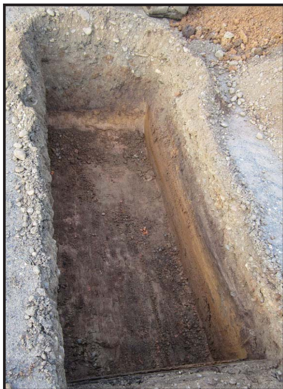
Figure 120. Trench 13 was dug with the excavator along Missionary Way SW.
