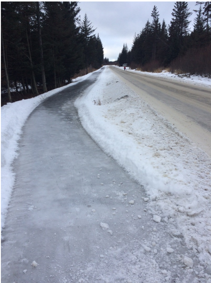
Spruceview Avenue Separated Sidewalk Unsanded
