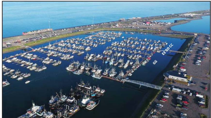
System 4 ramps to be replaced next.
