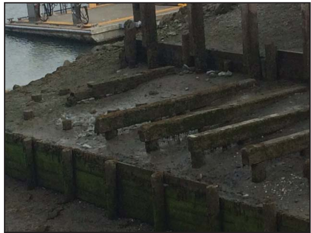
The Wood Grid in Homer’s Port and Harbor was originally built 40 years ago and accommodates vessels up to 59 feet with a 50 ton limit. Other than replacing the walkway in 2001, the wood grid has seen very little in terms of upgrades since.
