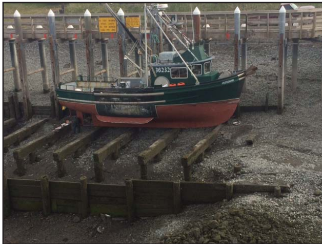
The Wood Grid in Homer’s Port and Harbor was originally built 40 years ago and accommodates vessels up to 59 feet with a 50 ton limit. Other than replacing the walkway in 2001, the wood grid has seen very little in terms of upgrades since.
