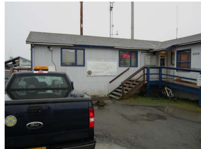
4. Harbormaster Office-East side.
