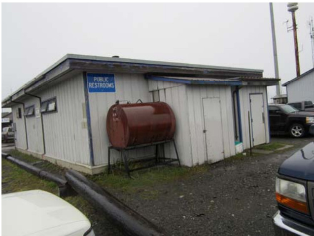
11. Restrooms-South and east side.
