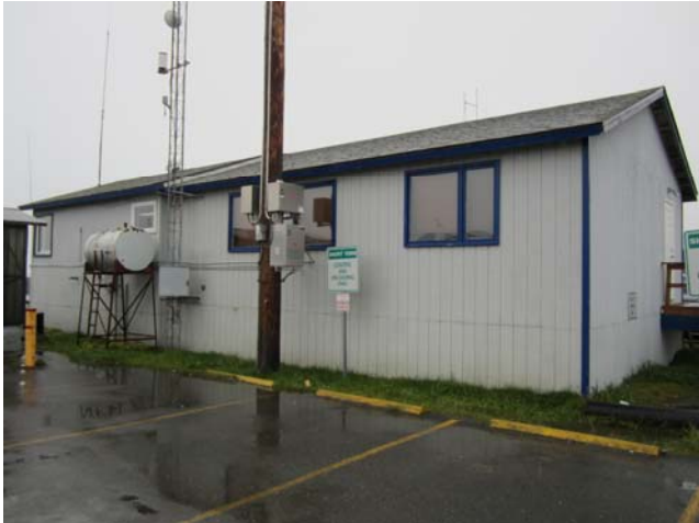
1. Harbormaster Office-West side
