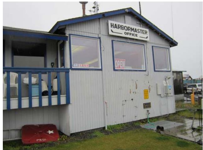
6. Harbormaster Office-North side.
