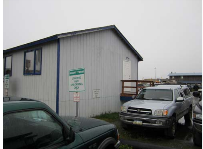
2. Harbormaster Office -West and South side.
