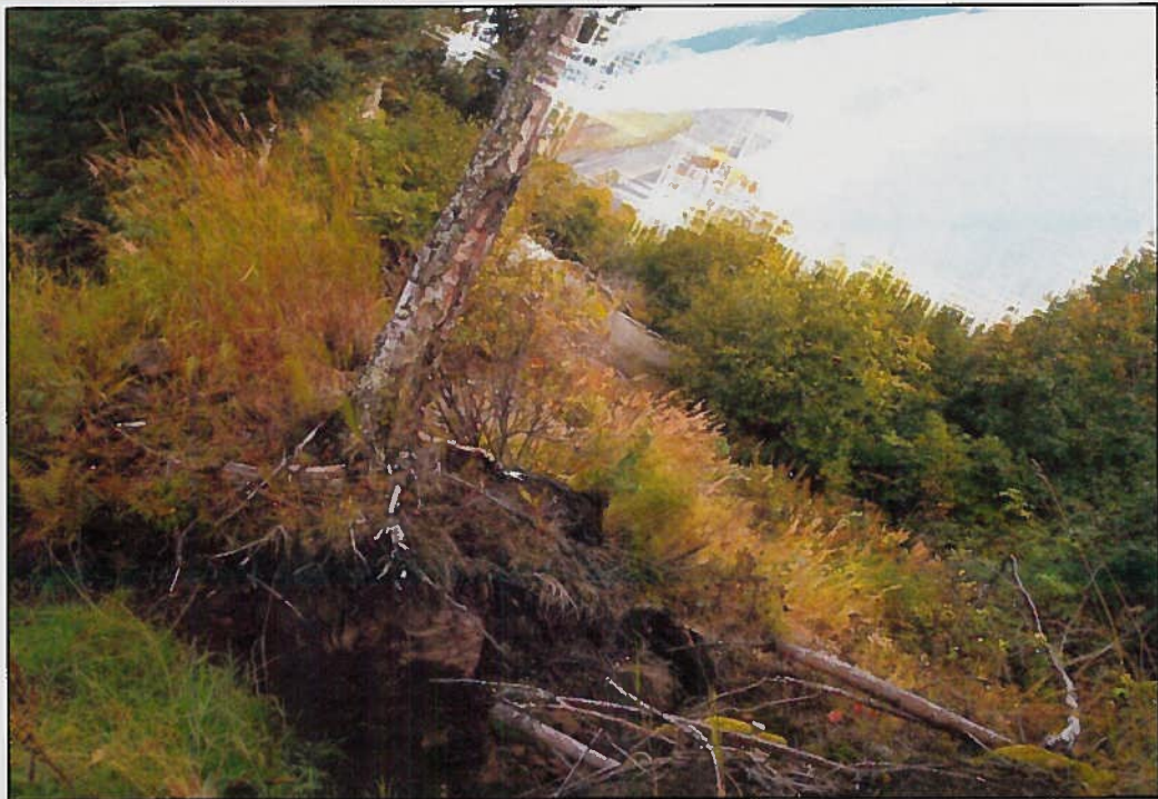
View SE over the edge of the bluff toward the Kachemak Bay beach.
