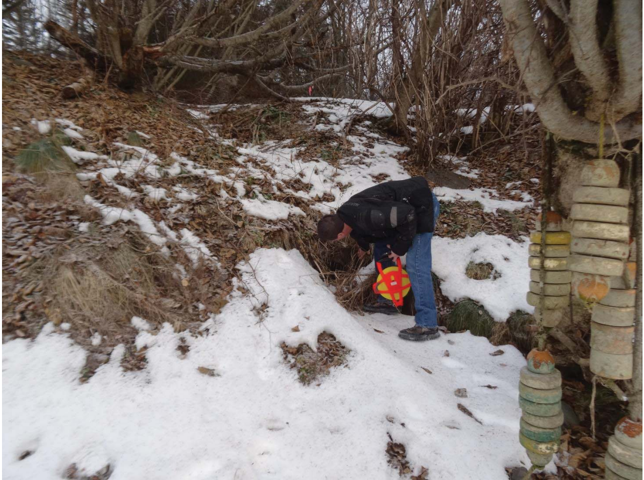
This photo looks north at the downstream end of the culvert that was removed.
