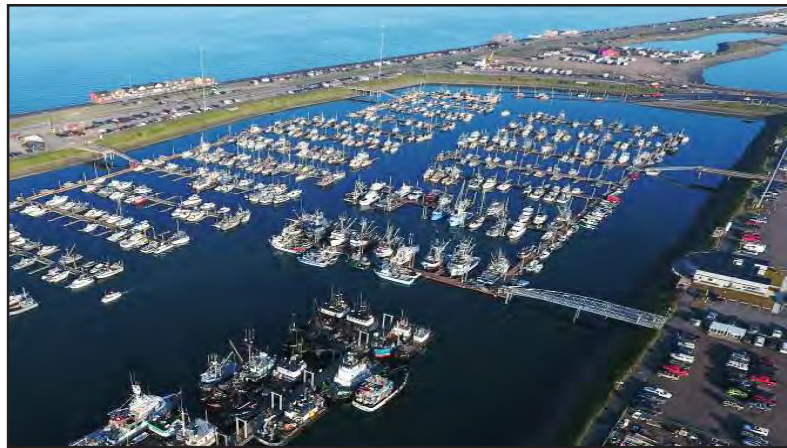
System 4 floats to be replaced.
