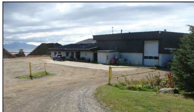
City of Homer existing Public Works facility.
