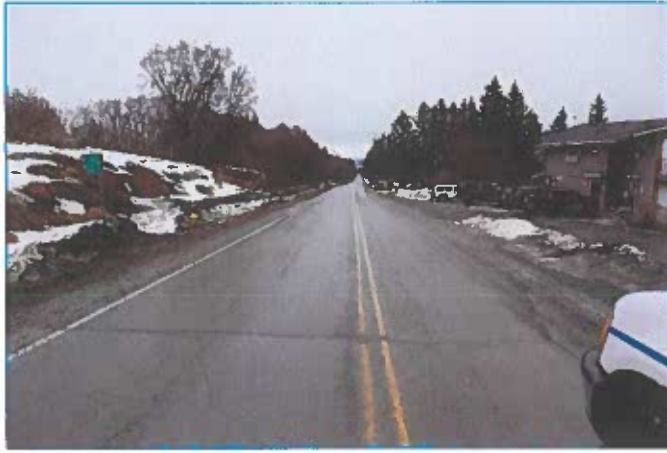
Fairview Ave looking east
