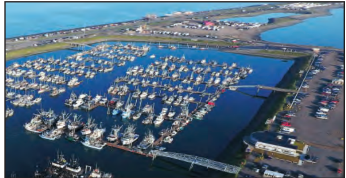
System 4 floats to be replaced.
