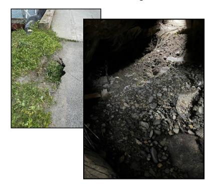
Working with Public Works and HDR we came up with a plan for what we hope will be a permanent solution. The affected area was excavated out. It was then built back with concrete blocks and heavy road fabric and re-enforced with concrete. The next step will be to asphalt and seal the surface. That will complete the necessary immediate repair and bring the Deep Water Dock approach up to full operational status.
