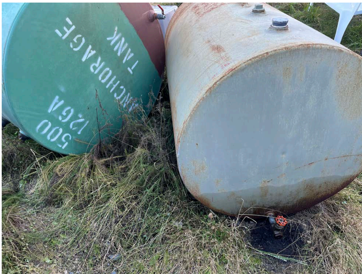
Photo __. This grey AST near the living quarters but not connected, does contain some heating fuel presumably and has a small leak around its valve.
