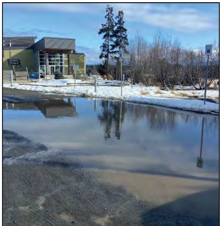
Poor drainage across Homer Public Library's sloped parking lot, especially during winter and spring freeze-thaw cycles, creates hazardous walking conditions.
