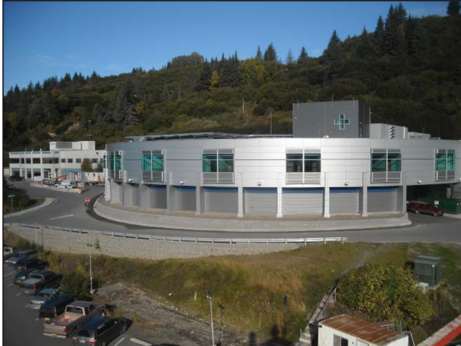
A hillside stability study on the slope behind the South Peninsula Hospital will yield recommendations on ways to minimize risk to the facility.
