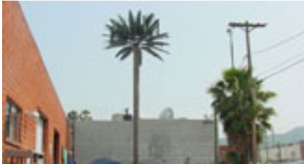
▣ Figure 9 Tower Camouflaged as Palm Tree
