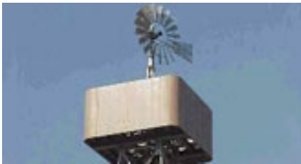
▣ Figure 11 Tower Camouflaged as Windmill
