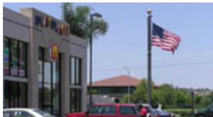
✚ Figure 6 Tower Disguised as Flag Pole
