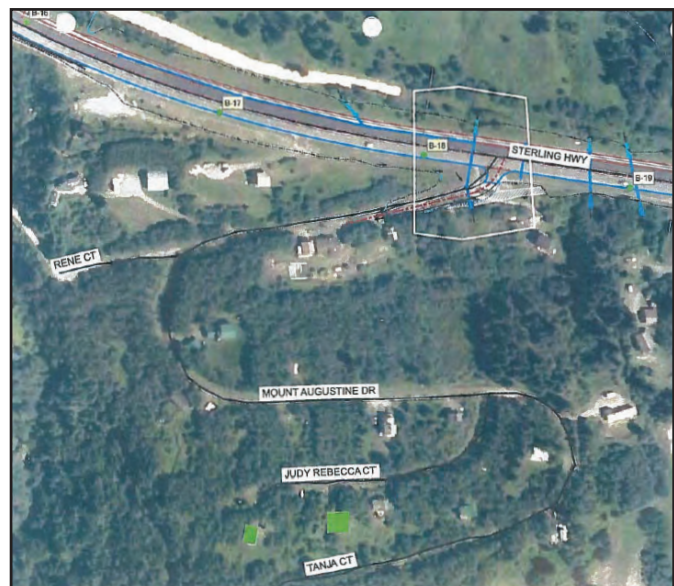
Aerial photo of the area downslope of the outfall from a Sterling Highway beehive collector.
