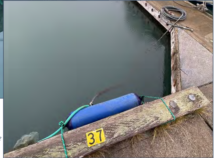
Figure 2.33: Water distribution, with location of valve at the far left (photo above) and hose coming up from under the float. Photo to right shows a hose from under the float to a 3-way connection, with one end going under the float and the other to a nearby slip, with a sprayer attachment.
