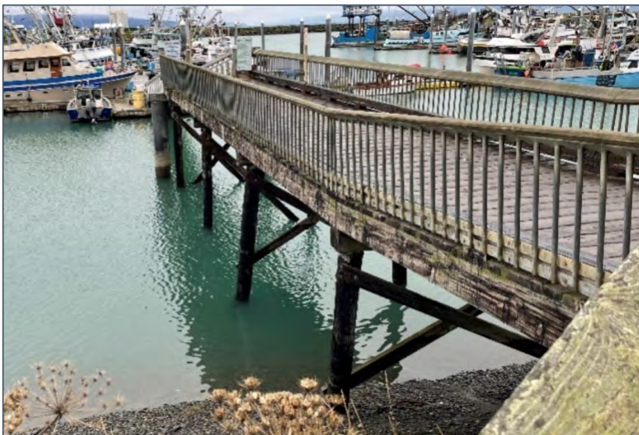
Figure 2.2: Ramp 1 timber pile supported trestle.
