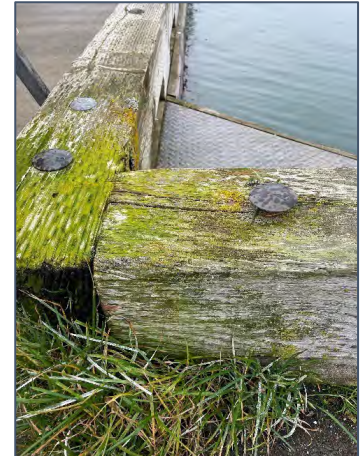
Figure 2.38: Deteriorated bullrails
