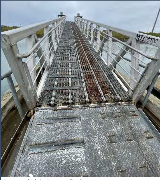
Figure 2.34: Ramp 5 aluminum gangway w steel floor grating.
