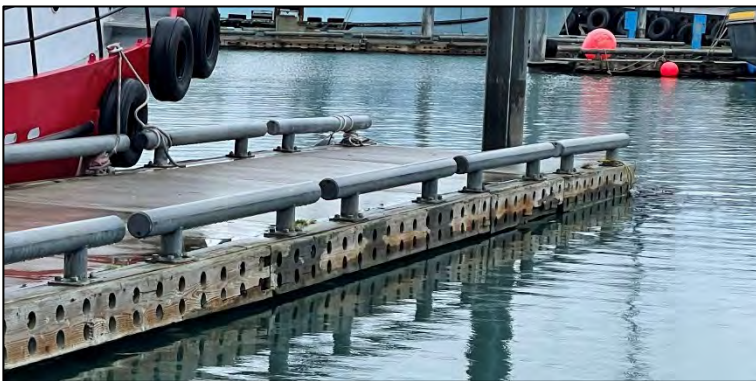
Figure 2.19: Concrete stall float with low freeboard, and in the water at the end.
