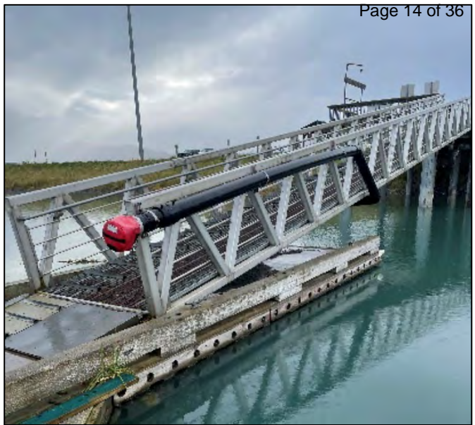
Figure 2.13: Fire system HDPE piping on Ramp 4.
