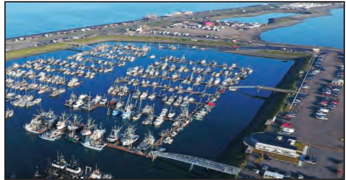
System 4 floats to be replaced.
