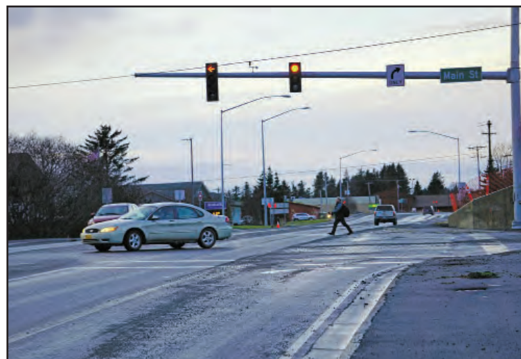
HAPP completes important sidewalk connections and installs high visibility crosswalks to improve non-motorized transportation and safety..
