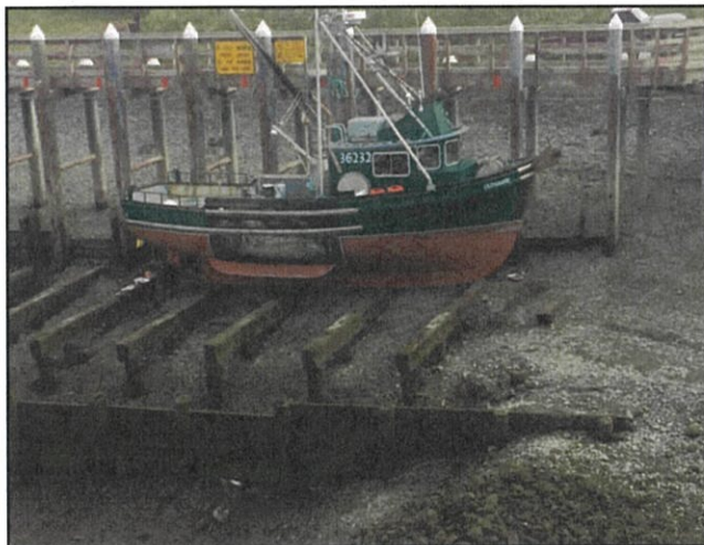
The Wood Grid in Homer’s Port and Harbor was originally built 40 years ago and accommodates vessels up to 59 feet with a 50 ton limit. Other than replacing the walkway in 2001, the wood grid has seen very little in terms of upgrades since.
