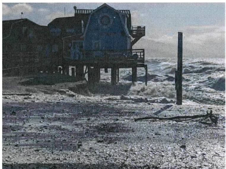
Example of recent active erosion on the Homer Spit.
