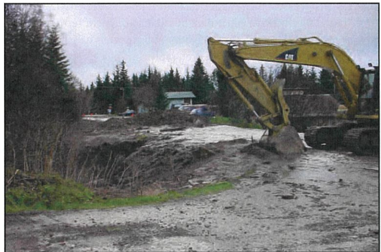
The Slope Stability Program utilizes nature based and low impact development techniques to mitigate erosional damage and protect water quality.
