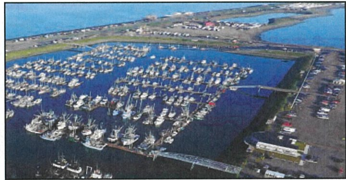
System 4 floats to be replaced.
