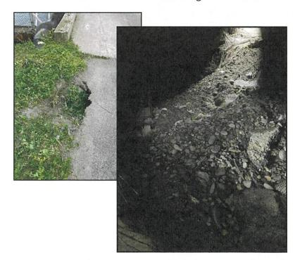
Working with Public Works and HDR we came up with a plan for what we hope will be a permanent solution. The affected area was excavated out. It was then built back with concrete blocks and heavy road fabric and re-enforced with concrete. The next step will be to asphalt and seal the surface. That will complete the necessary immediate repair and bring the Deep Water Dock approach up to full operational status.
