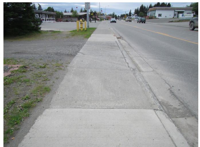
Figure 20: Driveway Entrance with Steep Cross Slope
