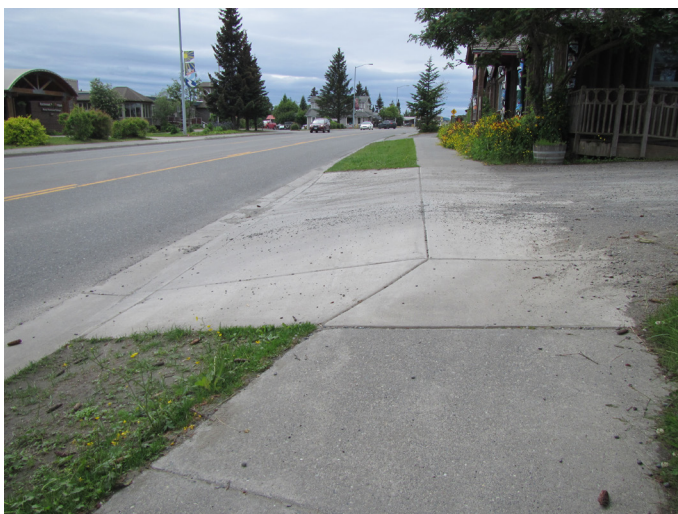
Figure 19: Driveway Entrance with Level Cross Slope
