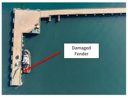
approximately 30,000 lbs. The fender system is designed to slide overtop of two pin piles that are driven into the seafloor and then are bolted to the dock face with brackets. Between the fender and dock are large rubber shock absorbers to assist with potential impact that can occur when a ship arrives at the berth.
