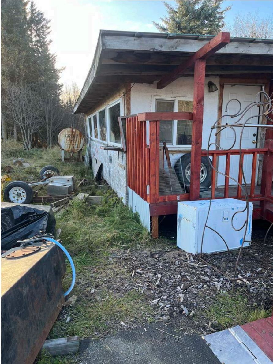
Photo -. AST associated with living quarters within the subject property scrapyard area.
