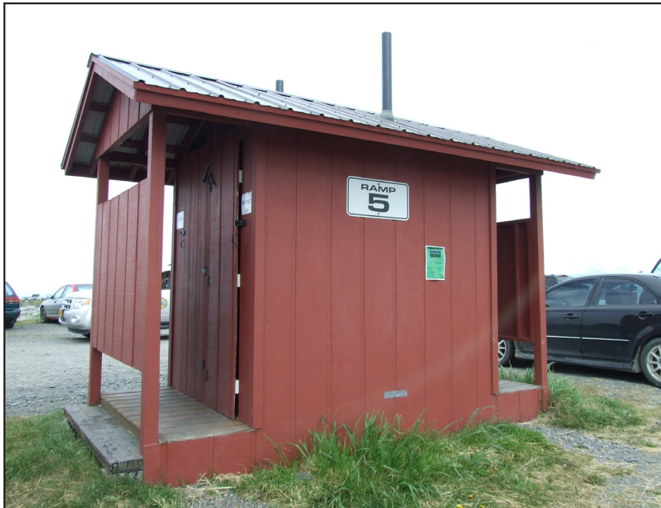
The outhouse at Ramp 5 is often the first time out of state visitors use an outhouse.
