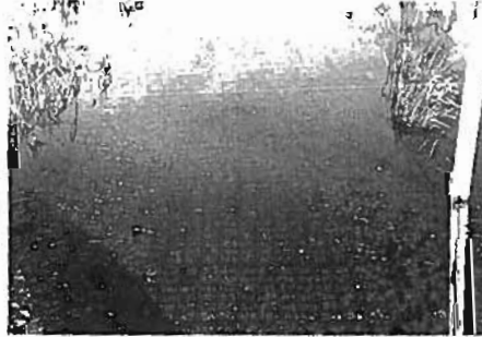
Porous pavement panels work underwater. Ballasted with small rock, filled with soil and planted, or otherwise anchored, panels function well underwater, making them highly suitable for drainage crossings. They spread the load enough to carry vehicles, including ATVs, without sinking into the wet soil below. Unlike currently available geocell, porous pavement panels do not need to be protected from sunlight.
