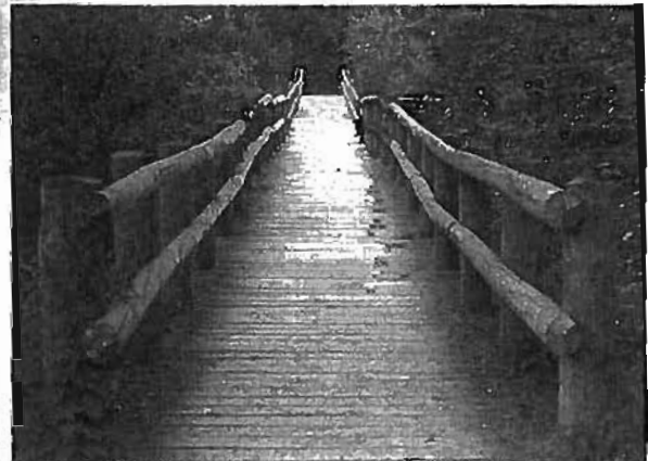
Thick timber posts, thinner rails, nonsquare end of posts and rails, and overlapping joints are rustic elements of this pedestrian bridge. The objective of rustic structures is to create a relaxed, natural character by avoiding straight or curvilinear lines, allowing rough materials to shape the details of how parts fit together.
