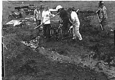
Paneled drainage crossing installation. Some panels (left) have flexible joints built in to enable them to contour to irregular treads. This photo illustrates a drainage crossing in an early stage. Grids can be left exposed or ballasted with soil or rock.
