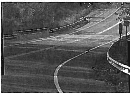
Bike route in narrower, slower speed roadway. Where space is limited and traffic speeds are 30 MPH, such as along this scenic byway, a minimum shoulder width of 4 feet would be adequate.
