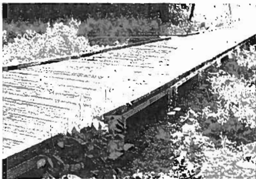
A growing number of premanufactured products are available for boardwalks and bridges. The main advantage to these products is cost and durability. As the photos illustrate, products include treated wood on steel frame (left), patented footings that require no excavation (middle), and various forms of plastic material that can be laid directly on the ground (right). Although these products have some advantages, their aesthetic qualities have to be carefully considered relative to the setting. On more remote or rustic trails, some products may be incongruent with the sense of place.
