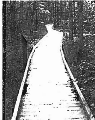
These boardwalks illustrate the range of possibilities and character. The two photos at left are associated with more remote trails where the idea is to simply get through an area without getting wet feet. This simple approach meets user expectations and there is no reason to do more. The two photos at right are associated with popular nature trails in state and regional parks, where the trail will appeal to a wider cross section of users, including those who are less ambulatory. Although more accommodating, these boardwalks still fit well into the settings.
