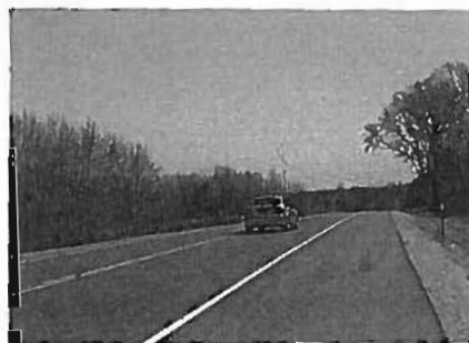
Bike route on wider, higher speed roadway. Once speeds get above 50 mph, a minimum 6 foot shoulder is recommended to provide reasonable separation between bicyclists and motor vehicles.
