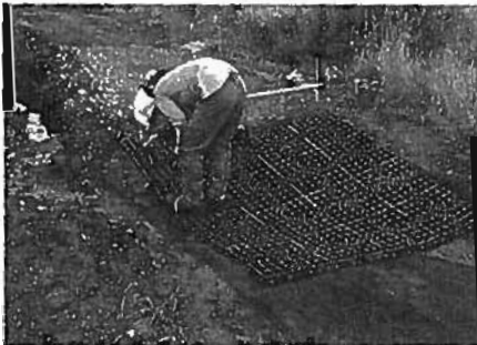
Green hardening. A major advantage of plastic porous pavement panels (top) is their ability to support vegetation. Each cell has a relatively large hole in the bottom through which vegetation can grow. This enables a drainage crossing to support plants even while serving as part of the trail.
