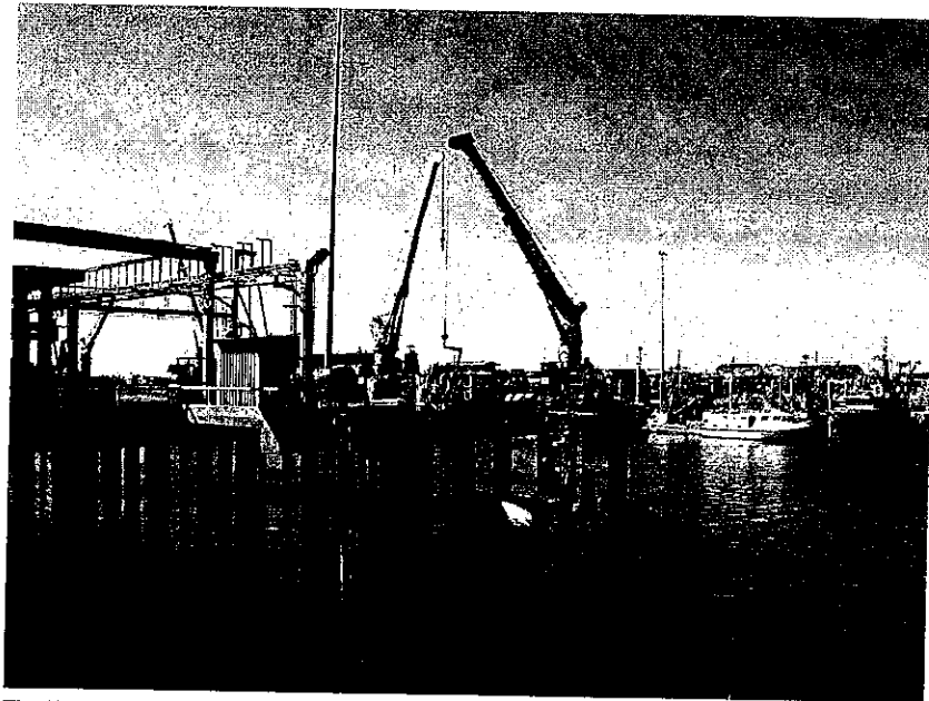
The Homer Fish Dock is one of the busiest places in the Homer harbor, but currently has no restroom facility.
