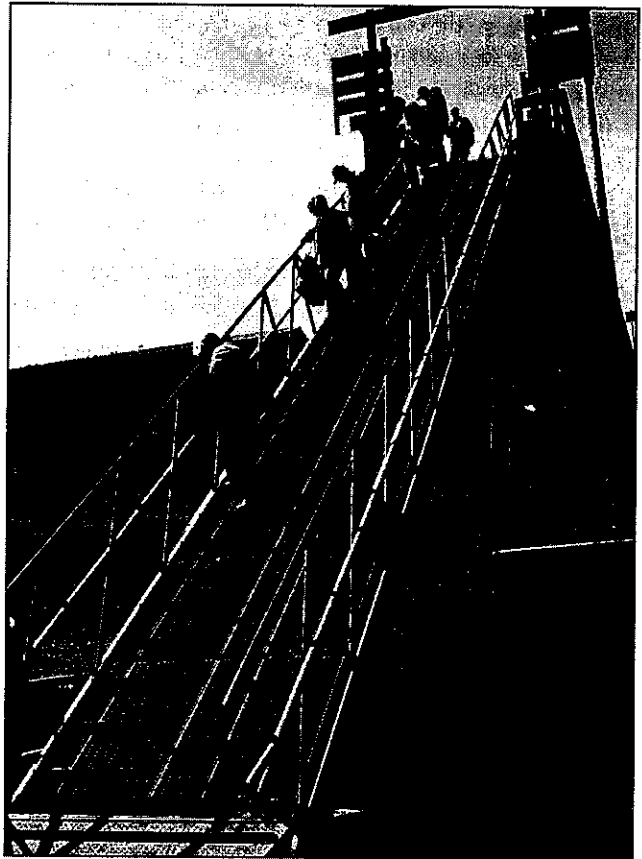
Ramp 3 is the most centrally located ramp in the Homer Harbor, but it is also the oldest and the most challenging to use at low tide. The old wooden approach to the ramp is also in need of replacement.
