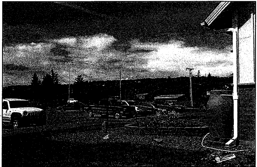
At various times of year, the Visitor Information Center parking lot is plagued by dirt, dust, mud, and potholes – sometimes all at once.
