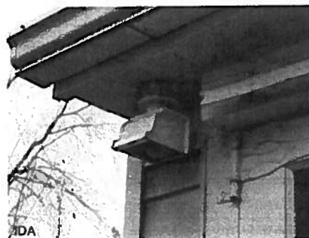
IDA Fixture shields can be made from household objects. This shield is made from a rain gutter.
