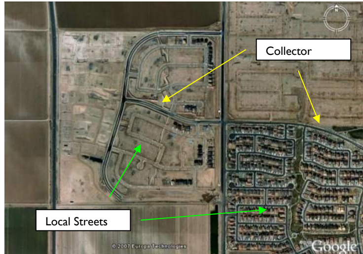
Figure 2: Collector Streets and Local Streets Constructed at the Same Time
