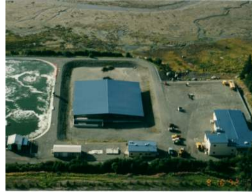
Sewer Treatment Plant (1990)
