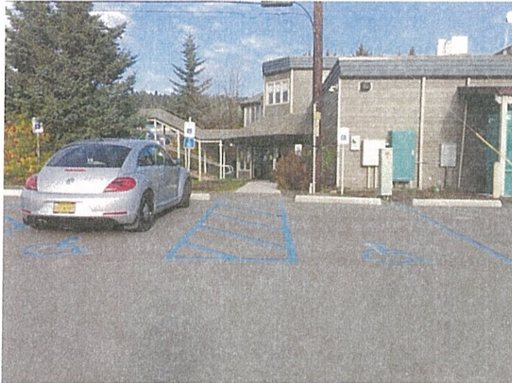
Access Aisle and secondary walkway to building entrance
