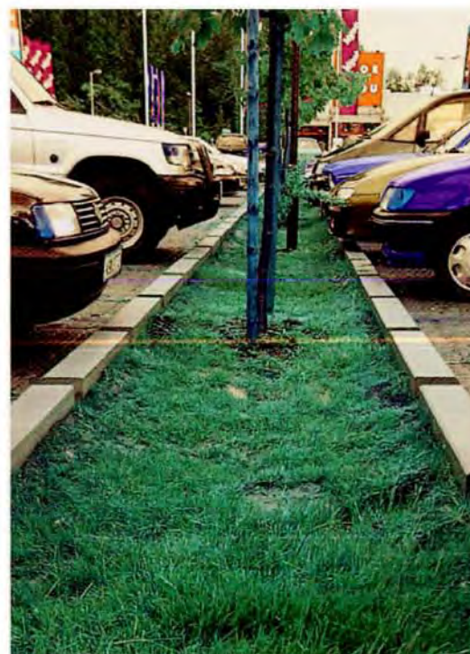
Planted swale separates parking stalls and collects stormwater.
