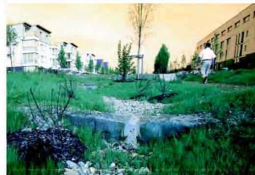
Planted bioswale near trail conveys stormwater.
