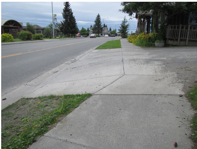
Figure 19: Driveway Entrance with Level Cross Slope
