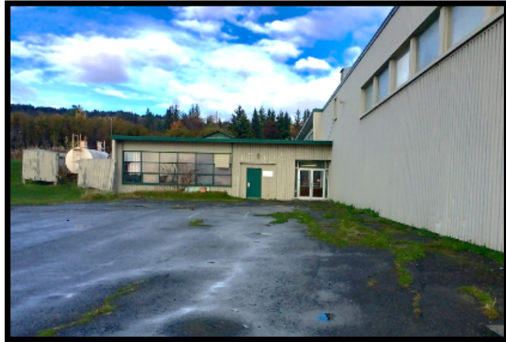
HERC-1 Lower Entrance Used to Access Gymnasium
