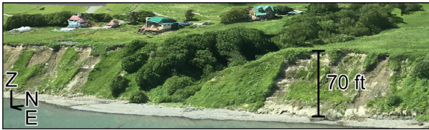
Figure 15. Looking west toward the grassy-to-exposed bluffs and a densely vegetated creek near East End Road in the oblique image-derived 3D model. Exposed slopes show groundwater flow.
