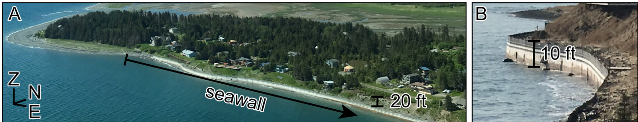
Figure 13. A. This 2019 photo looking northwest at Munson Point (left) shows the seawall protecting grassy and exposed bluffs. B. This closeup photo shows how water comes right up to the seawall and would surely undercut the bluffs.
