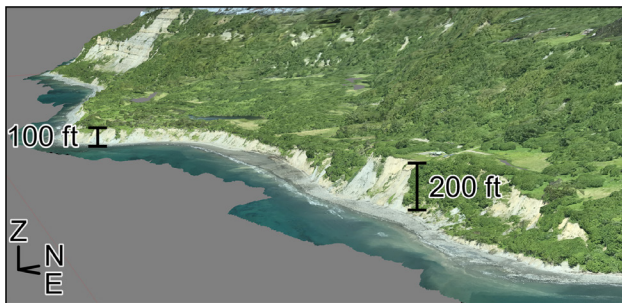
Figure 11. Looking northwest at the Bluff Point landslide area. The coastal bluffs are the seaward-most bluffs in this screenshot from our oblique image-derived 3D model. Unlike the larger bluffs in the background, these coastal bluffs are mostly unvegetated and experience significant erosion.
