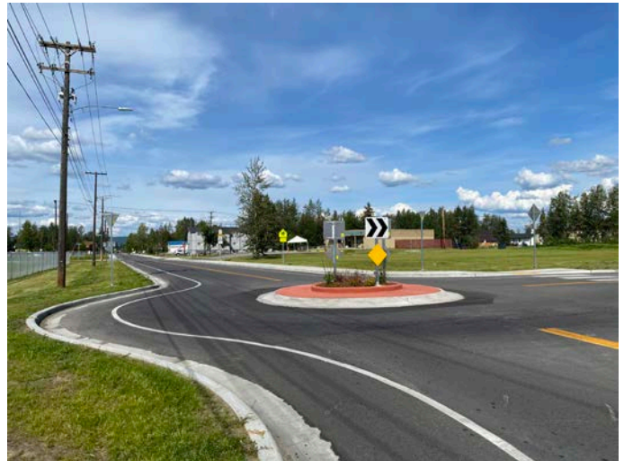
Figure 25: Traffic Circle on Gillam Way in Fairbanks
