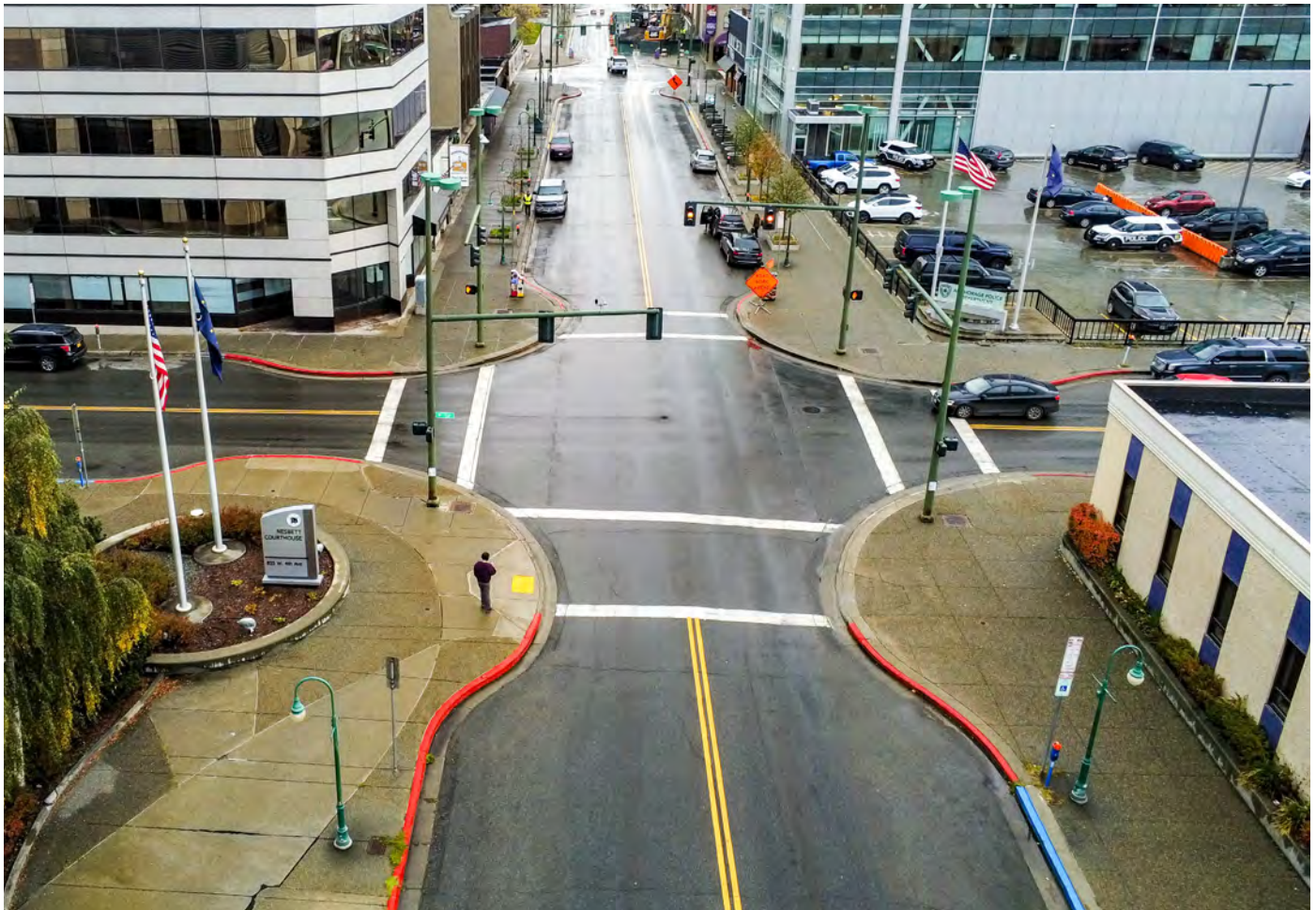
Figure 24: Curb Bulb-outs in Downtown Anchorage, Alaska
