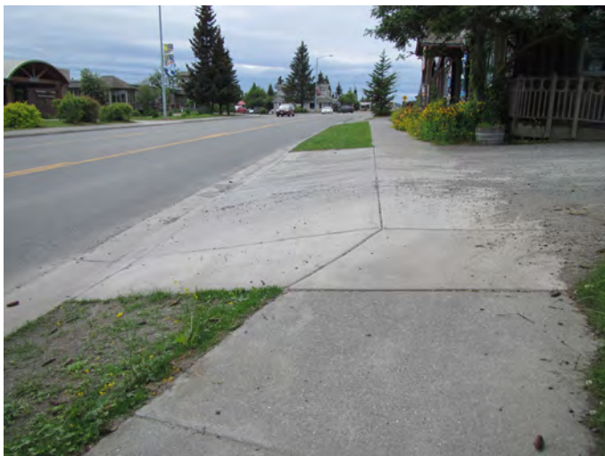
Figure 19: Driveway Entrance with Level Cross Slope
