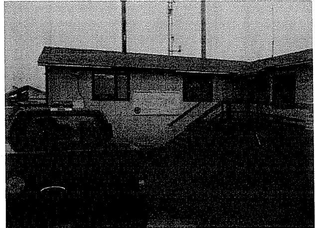
4. Harbormaster Office-East side.
