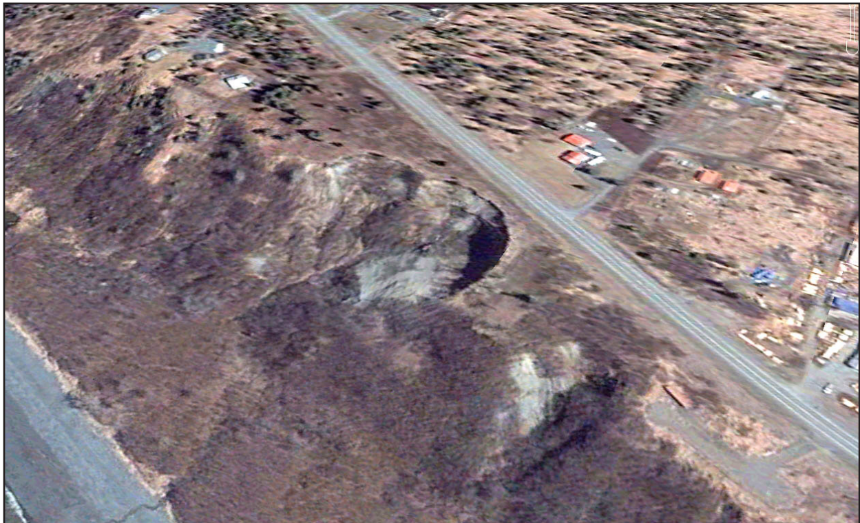
As seen in this aerial image, the eroding edge of the bluff is now only 30 feet away from the Sterling Highway at a section just north of Anchor Point.
