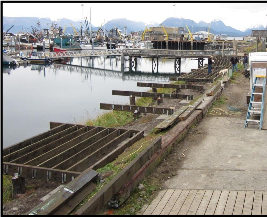
Harbor Boardwalk Reconstruction
