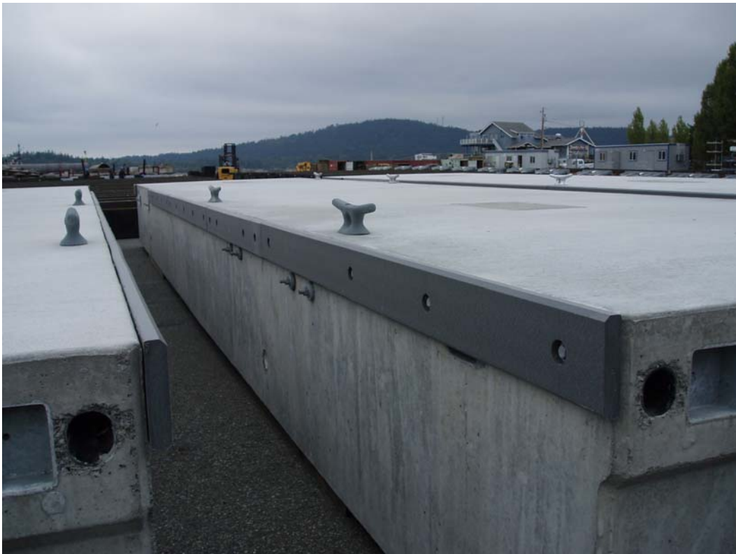
Figure 3-2: Concrete Float Units
