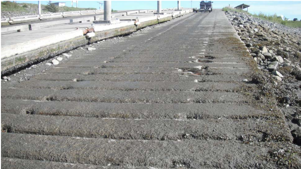
Figure 1-2: Existing Concrete Launch Planks
