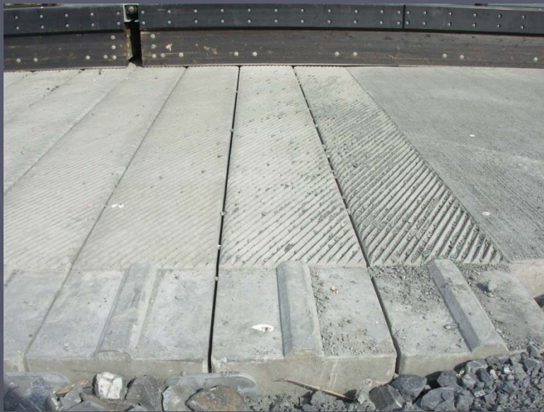
Ramp panels with V-grooves and rumble strip
