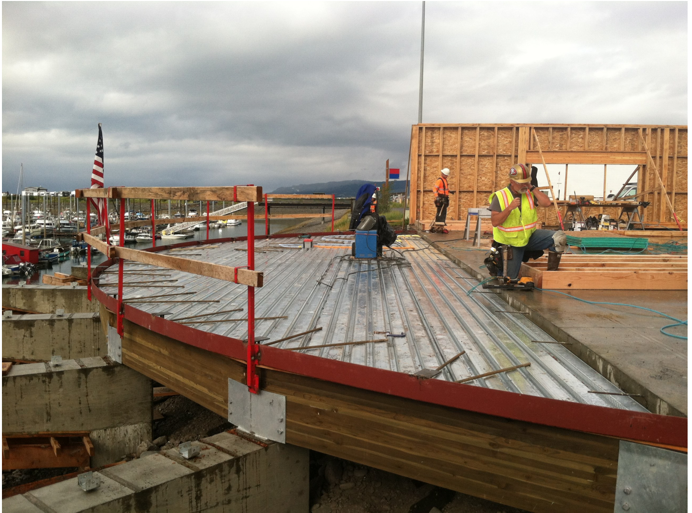
New harbormaster office, under construction
