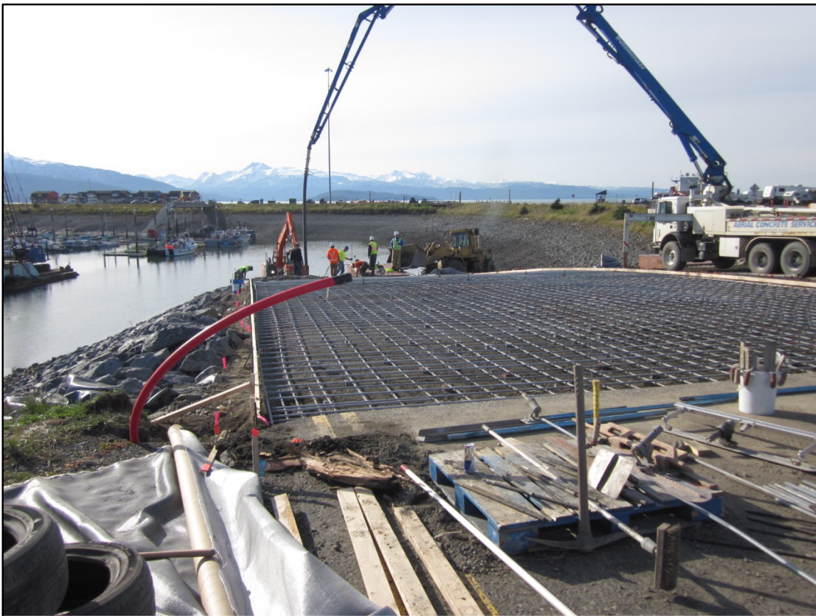
Load & Launch Ramp construction
