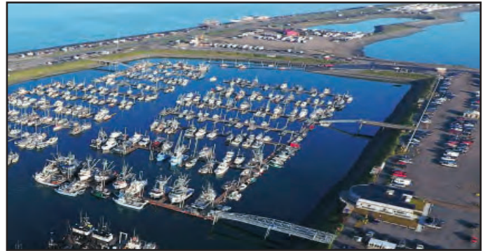
System 4 floats to be replaced.
